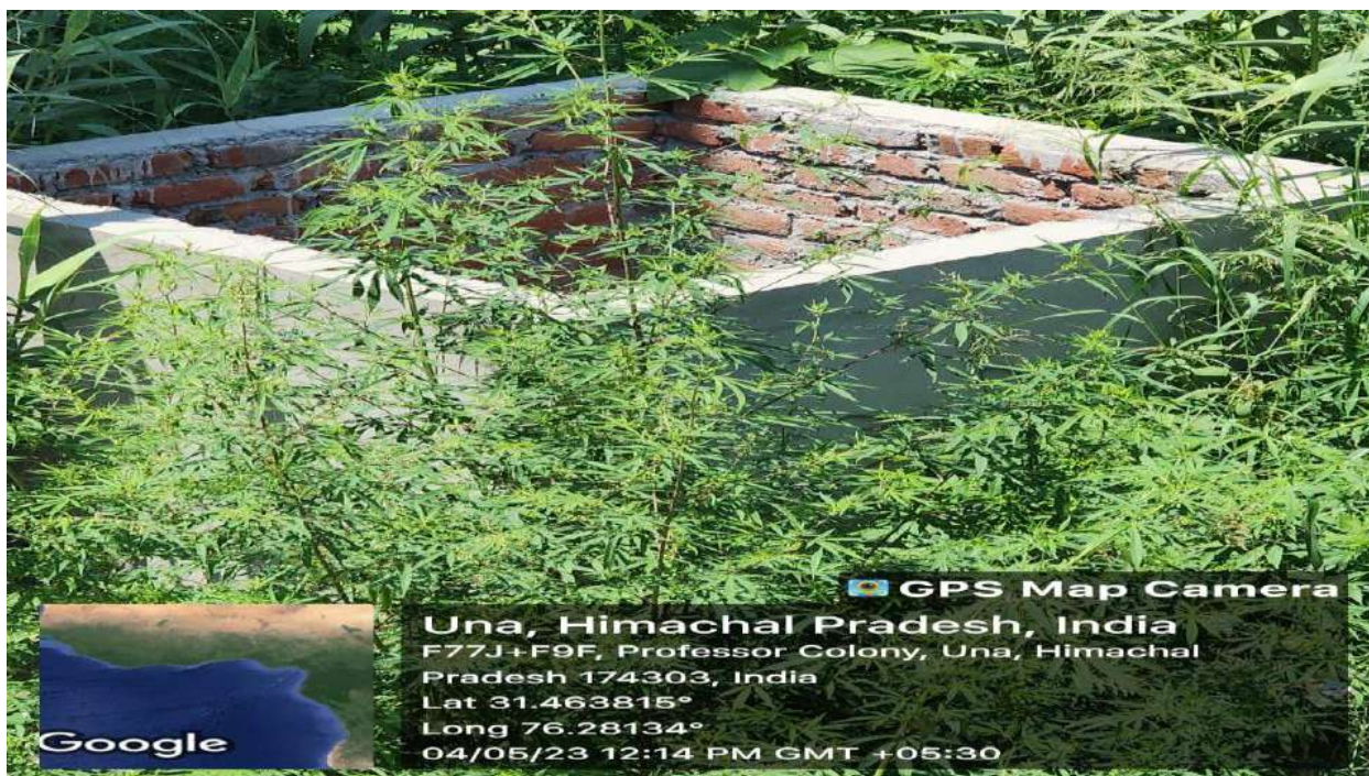
Figure 4 Pit to collect solid waste.
